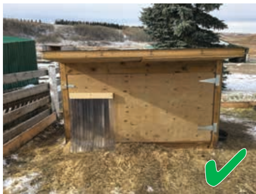
2. Shelter with door access.
