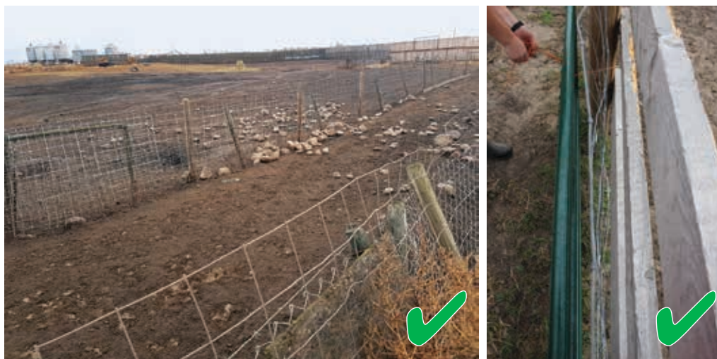
1. High double fence lines with space in between fences to prevent nose to nose contact with wildlife. 2. Strong double fencing with hog panels and hog fencing buried into the ground. Photos: Dr. Kelsey Gray
